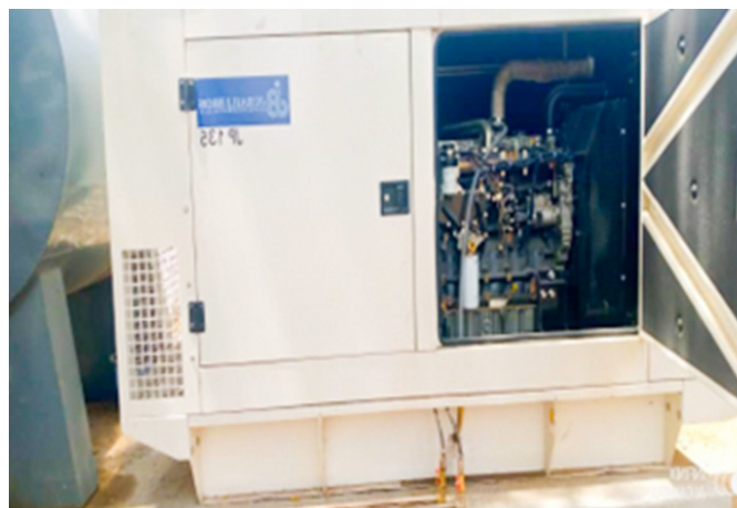
Photo 2: Industrial diesel generator installed in one of the supported PCR labs.
