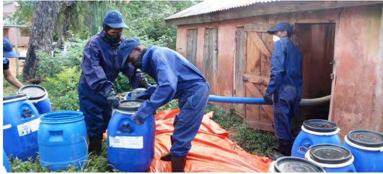
Trained workers use the Gulper to extract sludge from a row of pit latrines at an office building in Ambositra as part of WASHplus's pilot project to test fecal sludge removal tools and business models.
