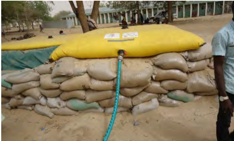
Figure 8: Overhead water tanks supplying one of the camps
